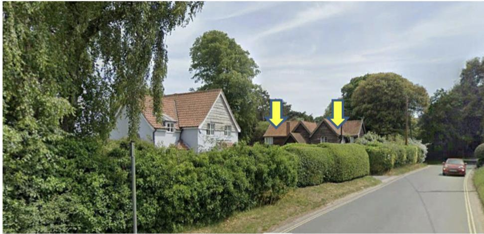
Position of solar panels
