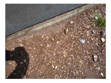
Surface is lifting. Recommend rearrange, re-glue and fill gaps and joints as necessary - Low risk.
