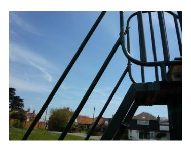
NB Although not part of EN1176 – the slide surface faces south and may suffer from solar gain and get hot during the summer – Recommend monitor –Low risk.
