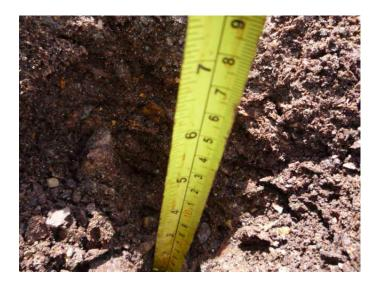
Trip zones found at edge of surface. Recommend build up ground levels to remove trip hazard (see above) - Low to Medium risk.
