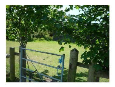
Access –Recommend removed damaged log under pedestrian gate, which is a trip hazard –Low to Medium risk.
