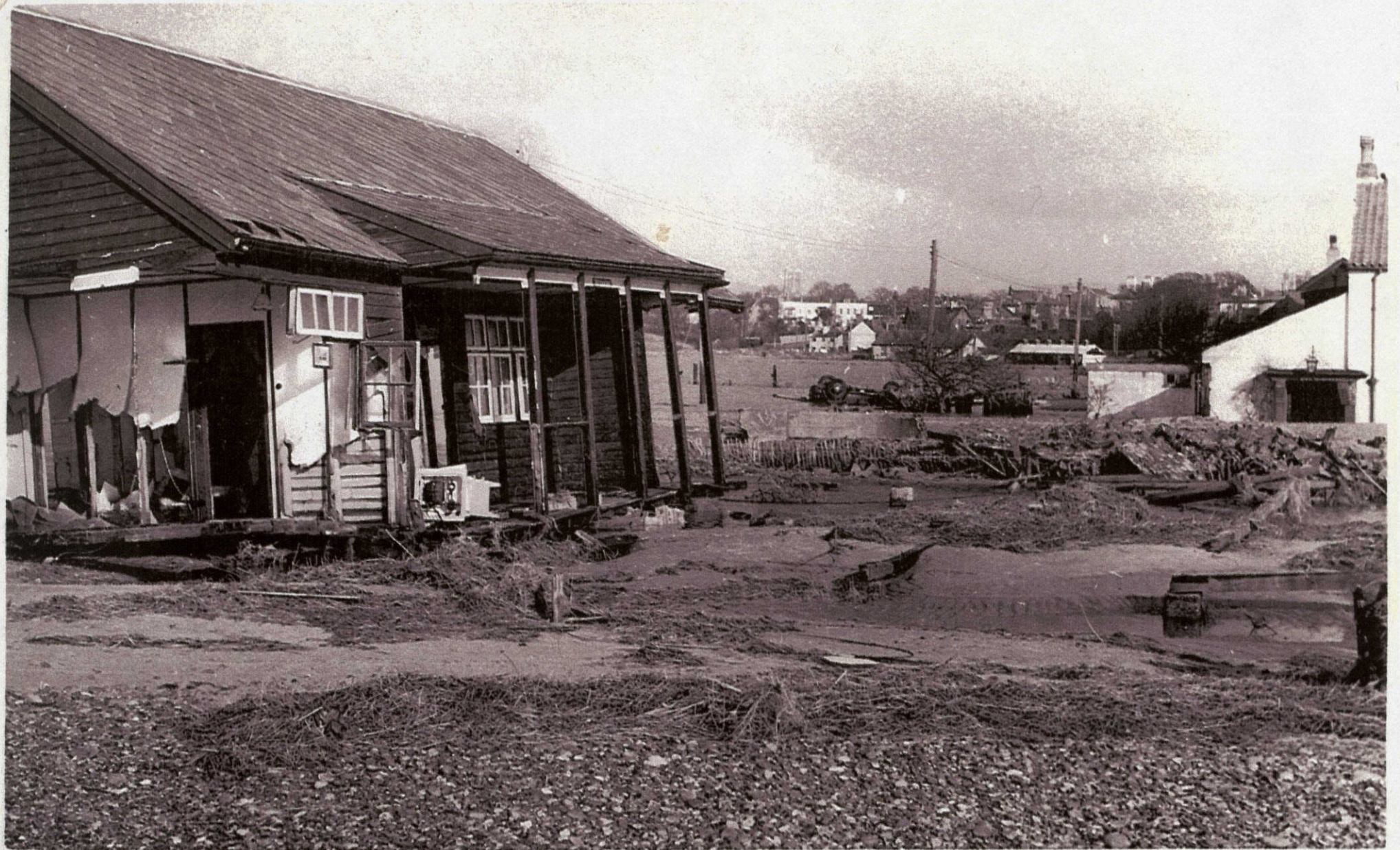
Close up of the destruction of one of the Bungalows.
