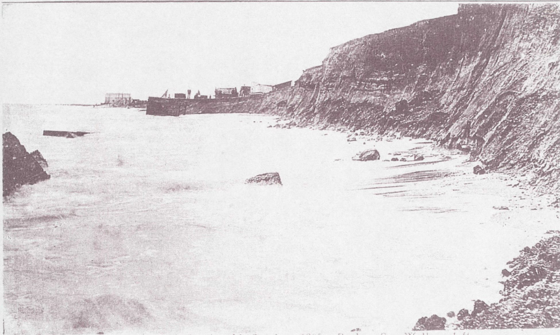
Damage caused at Gunhill, Southwold, October, 1905. Broken Sea Wall on left
