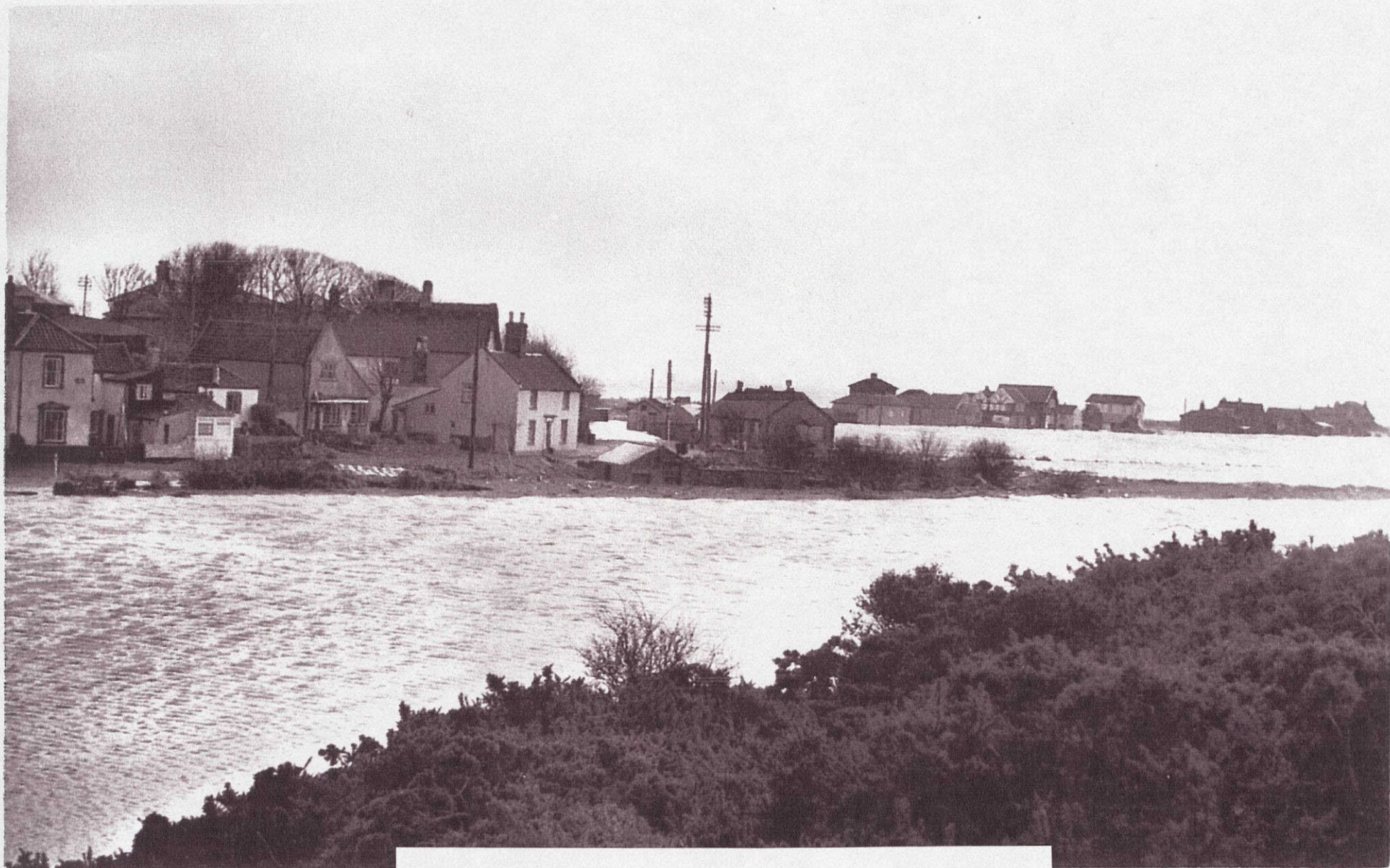
The lower end of South Green, the sewerage pumping station roof shows above the tide washings, looking to Ferry Road.
