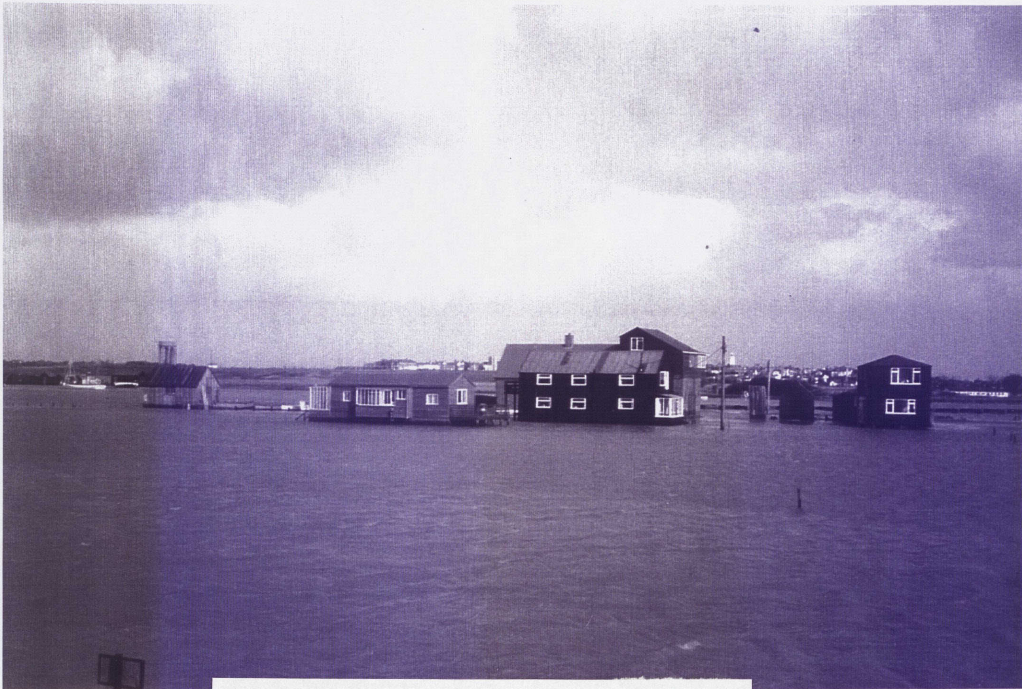
One of our regular floods "East Point" is the building on the right of the picture.
